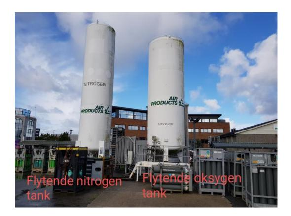
5.3 In the event of a leak from the storage tank with Oxygen, this will also immediately start evaporation and go up into the atmosphere. However, as Oxygen is oxidizing, it is highly flammable and will significantly aggravate any fire.
